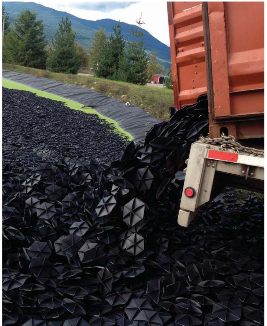
Truckload of Hexa-Covers added to the Nakusp lagoon.
