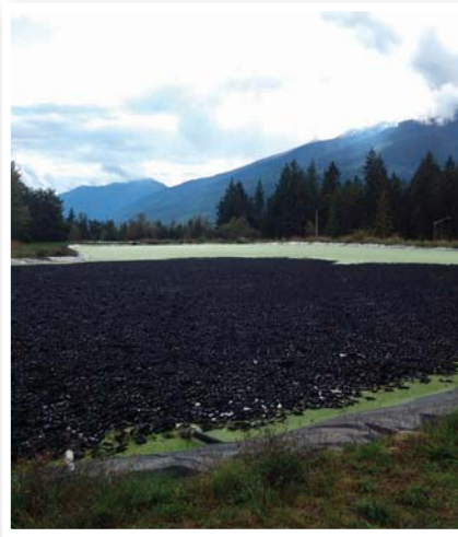
103,600 Hexa-Cover tiles were placed into the lagoon.
